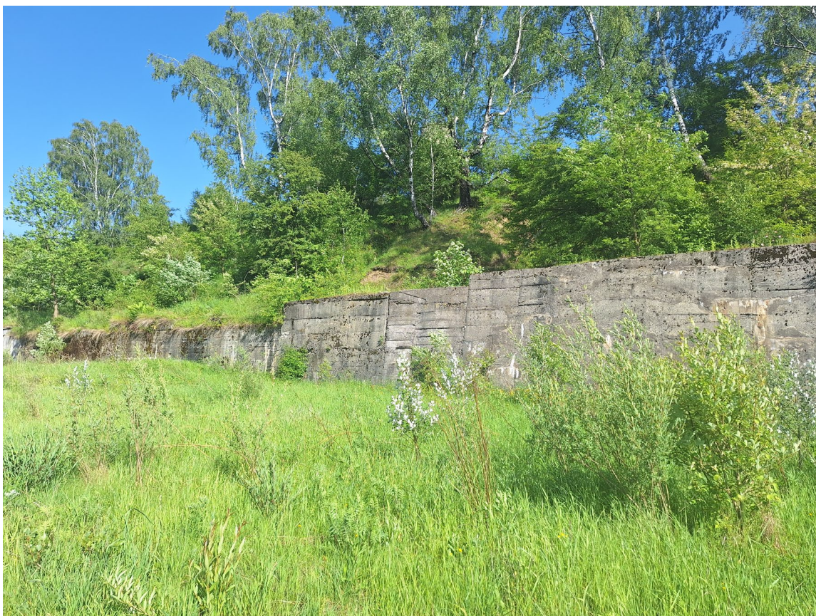
Zid sprijin taluz superior
